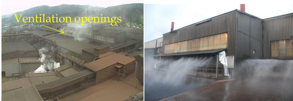
Figure 3a: Overview of furnace building ventilation openings. b: Water sprays over ventilation openings
