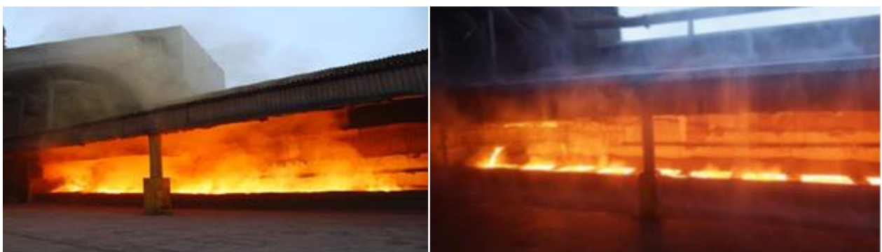
Figure 4: MCFeMn casting bed showing fume emissions over the roof without (left) and with water sprays (right)
